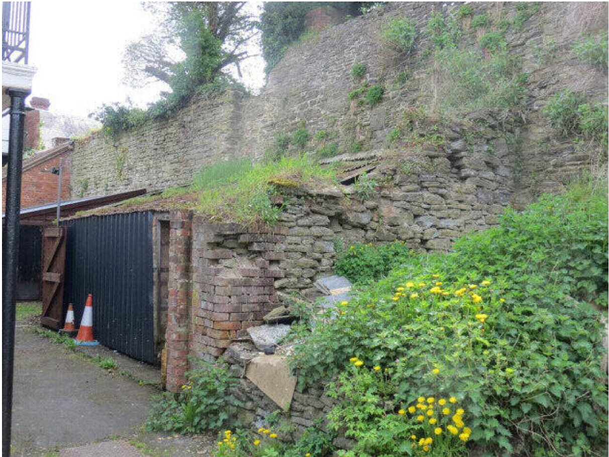
Photograph 11: Stone butress at junction with Compasses courtyard area (2018)
