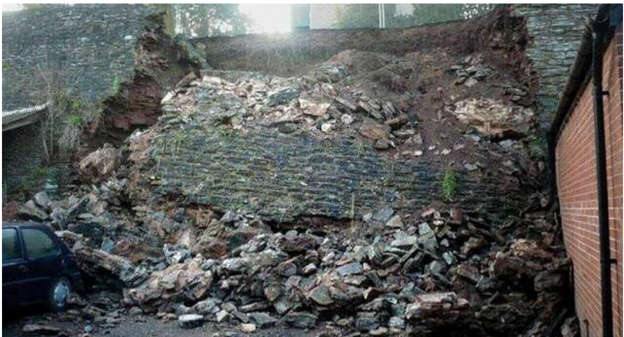
Photograph 2: Soon after collapse in February 2013
