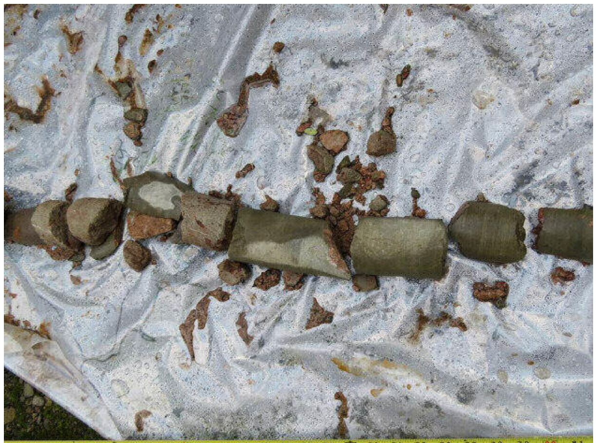
Photograph 27: Close up of core through wall to west end
