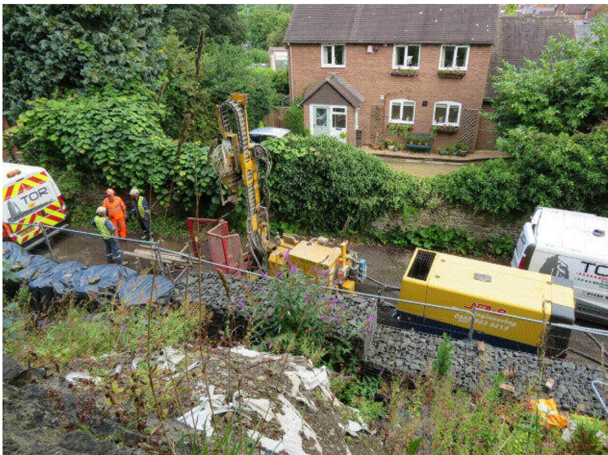
Photograph 29: View looking down on road to north of wall during investigations
