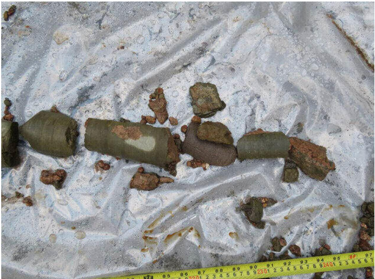
Photograph 26: Close up of core through wall to west end
