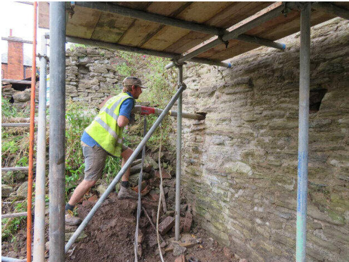
Photograph 24: Additional core hole P7 from initial investigations
