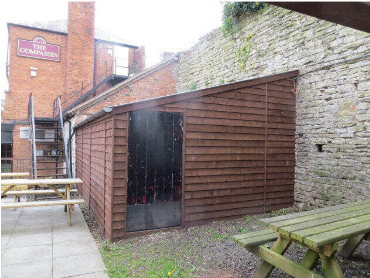
Photograph 13: Shed against wall in Compasses courtyard area (2018)
