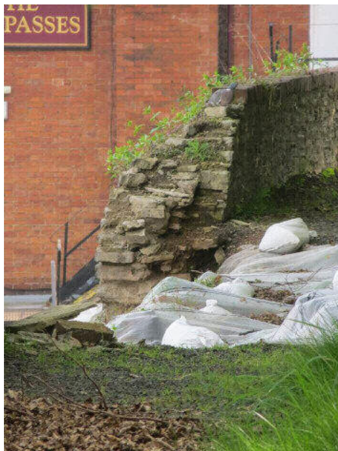
Photograph 6: View of end of existing wall with rubble core matrix apparent (2018)
