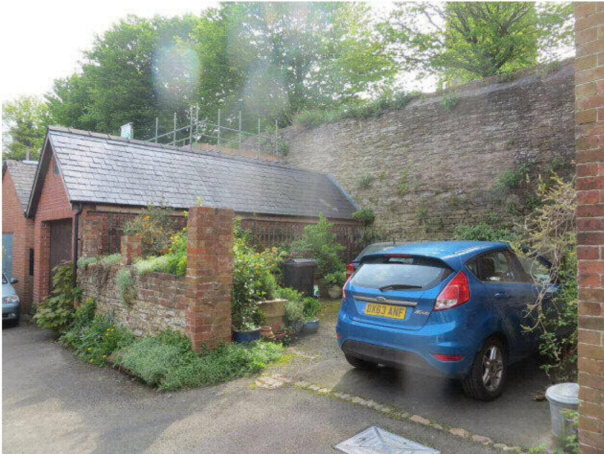
Photograph 7: Wall with two garages to St Leonard's House acting as buttresses (2018)
