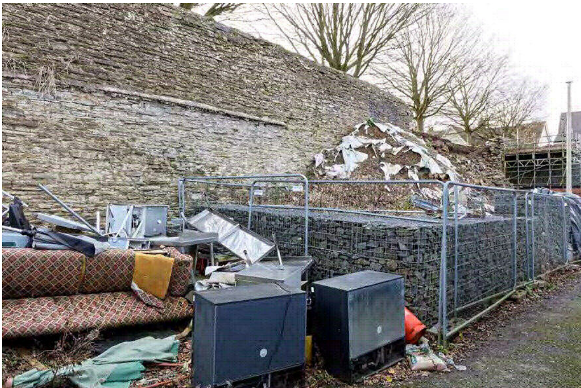
Plate 17 Central part of churchyard retaining wall (James Brennan Associates)
