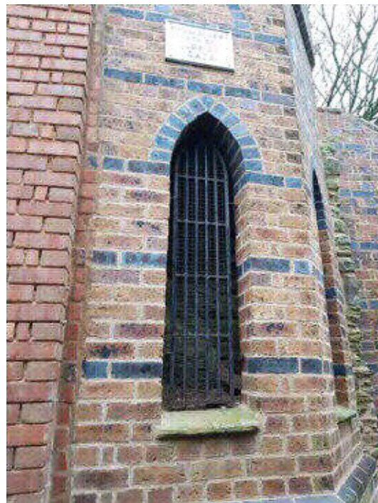
Plate 3 Remains of Linney Gate, with a brick structure
