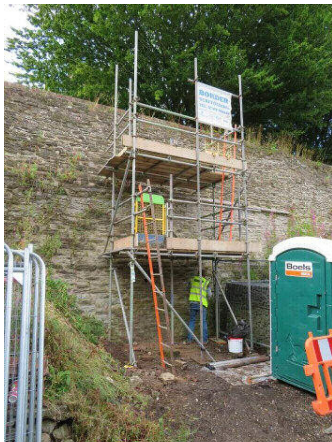
Photograph 23: Scaffold erected for west set of wall cores
