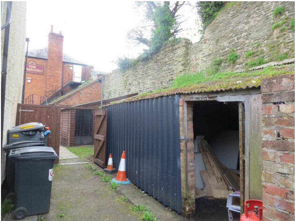
Photograph 13: Lean to against wall (2018)
